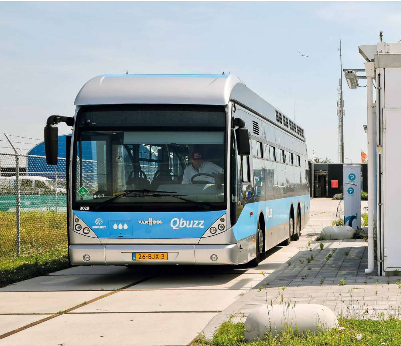
Hydrogen fueling station Delfzijl
