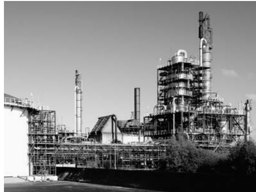
Chemical site Delfzijl: green chemicals production
