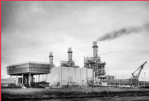
Magnum power plant, to be fueled by green ammonia-hydrogen
