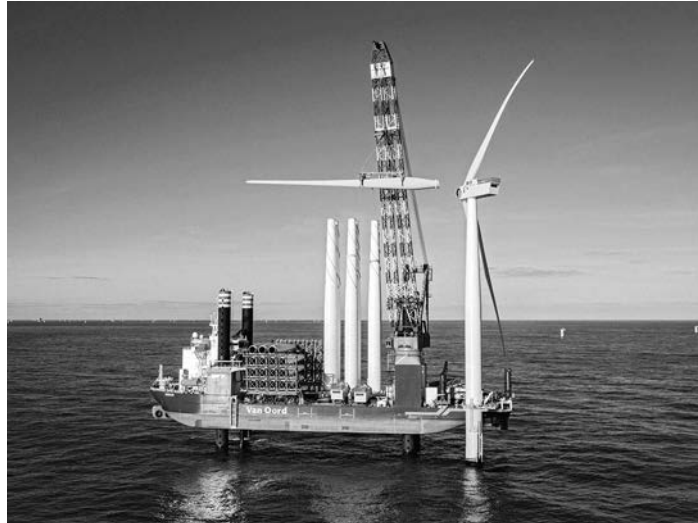
Gemini offshore wind farm, under construction
